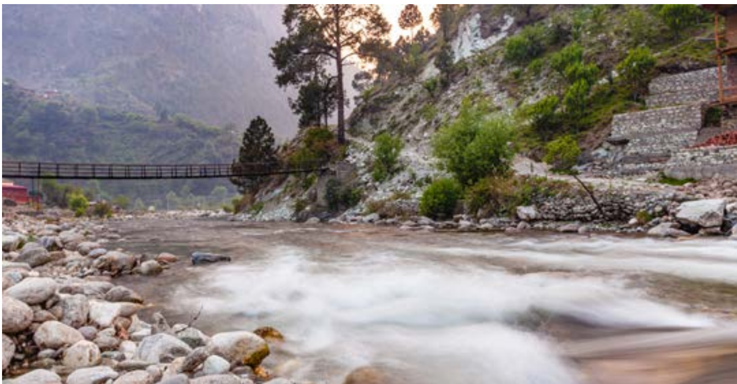
The Bridge over Tirthan River - Raunak Khubani
